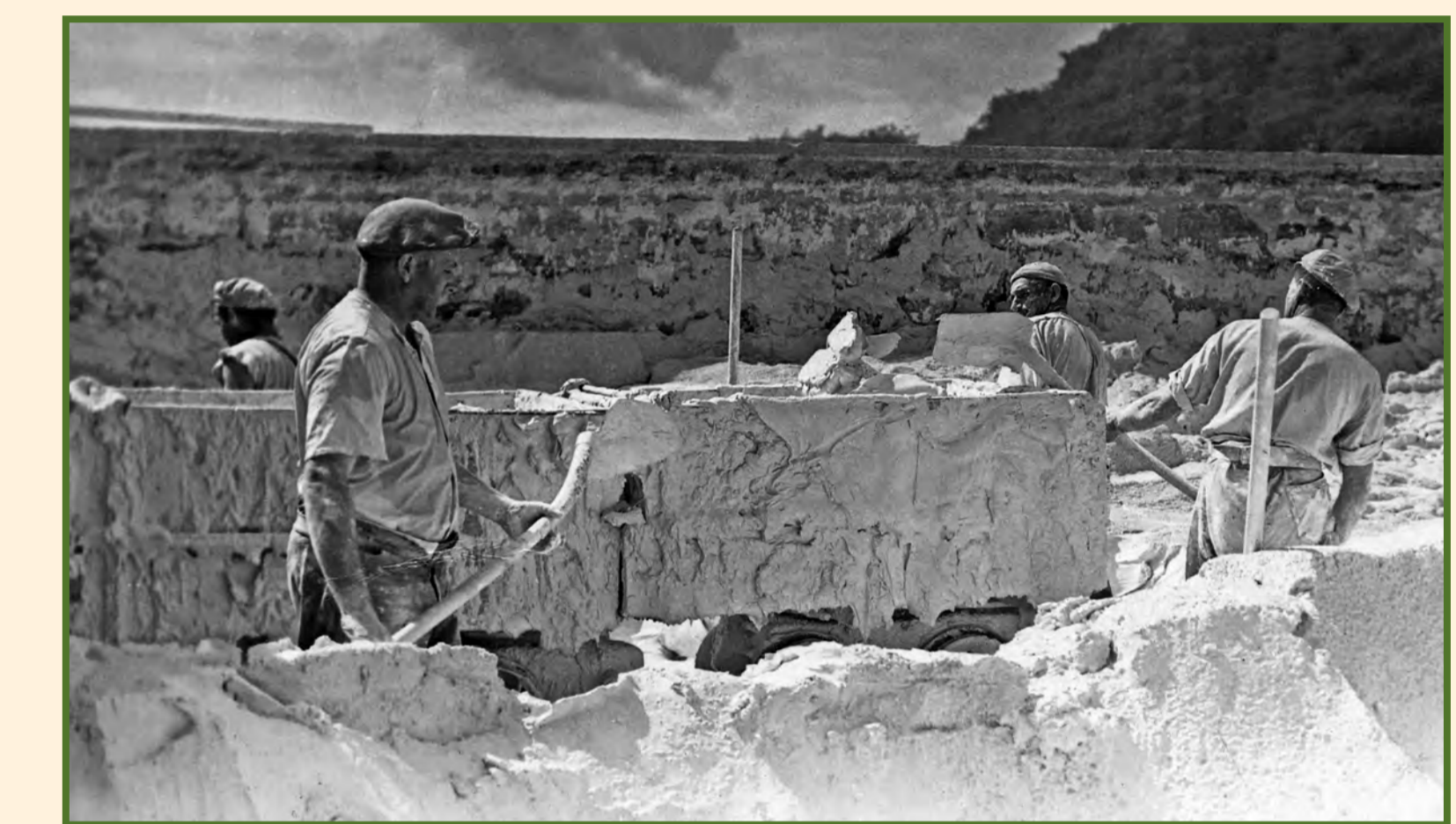
Clayworkers emptying a clay settling tank at Pontois Mill in the early twentieth century
