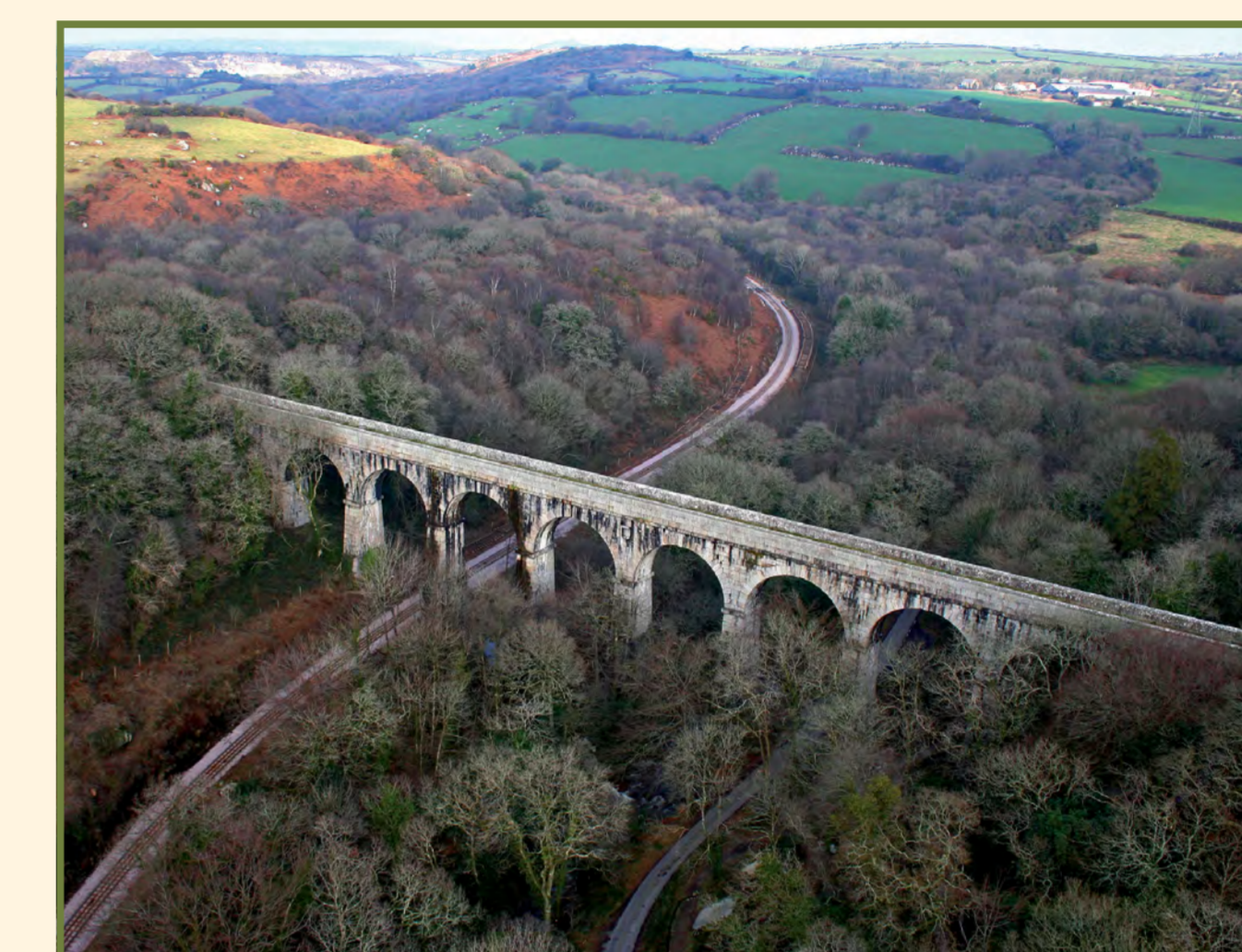
Aerial view of Treffry Viaduct, built 1839-1842, to enable rail access to the china clay and stone reserves in the Hensbarrow district and to link with Treffry's harbour at Newquay. The Viaduct also carried water to power the Carmears Inclined Plane, after which it flowed into the Fowey Consols Mine leat to provide additional water essential for the mine's operations
